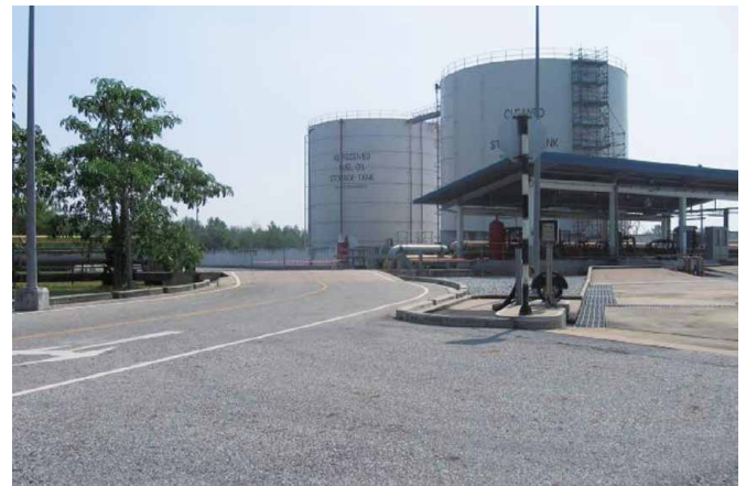
Bang Bo Power Plant
