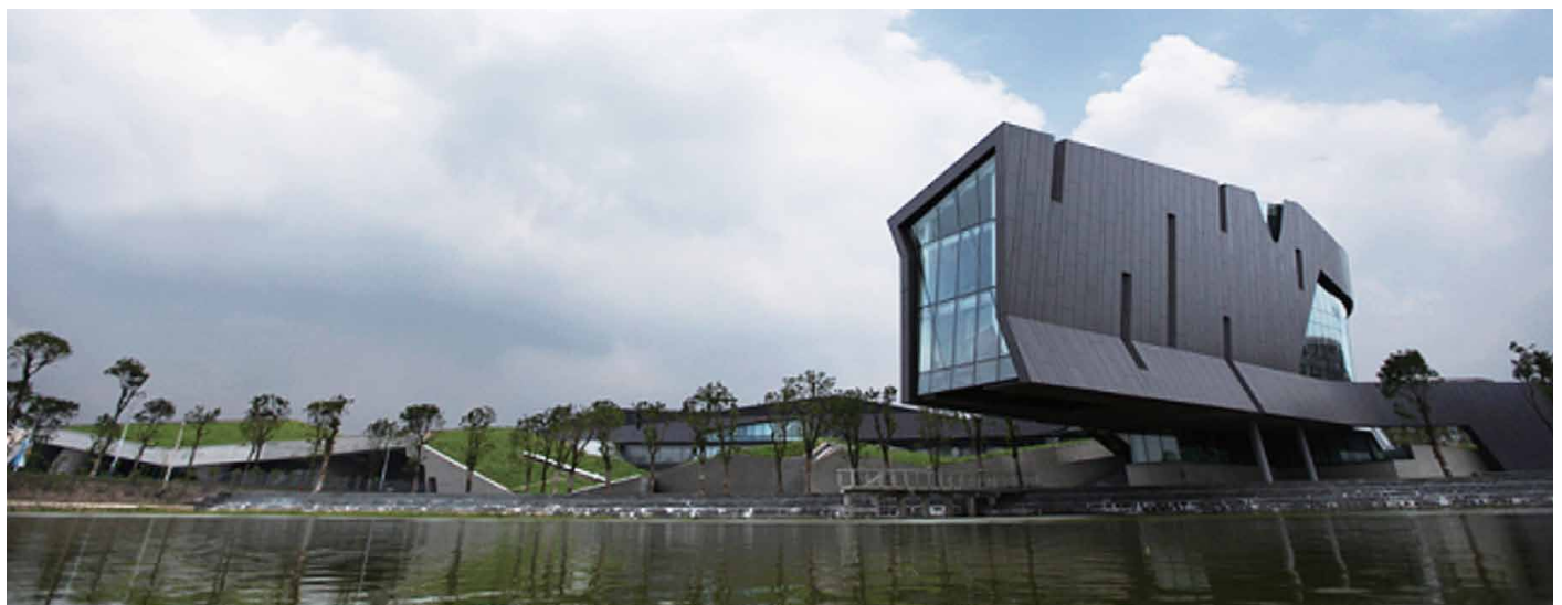
Giant Group Pharmaceutical Campus and its Green Roof Design
