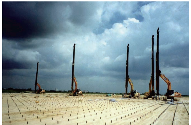
Installation of 40,000,000 m PVD with depth of 35 m
