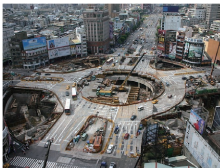
Largest circular excavation with diameter of 140 m in Taiwan
