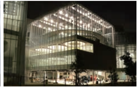
Metal Expanded Mesh and Low-energy Glass Reduce Heat Load and Energy Consumption
