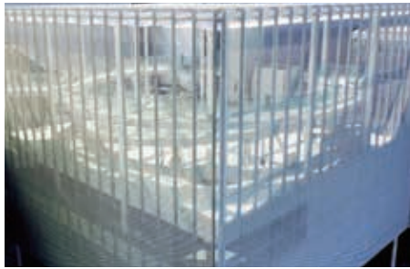
Metal Expanded Mesh and Low-energy Glass Reduce Heat Load and Energy Consumption
