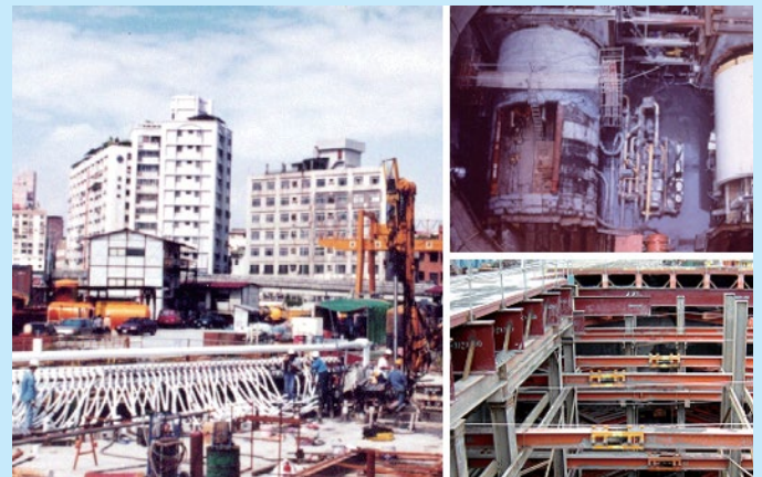
Frozen Method for Soil Improvement (left); Shield Machine (upper right); Deep excavation of a MRT station (lower right)
